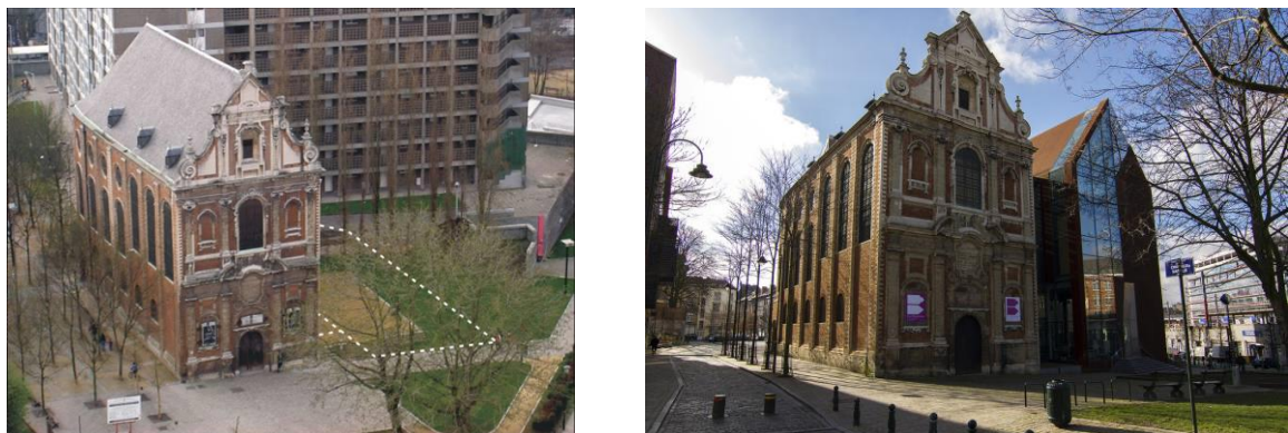
Figure 15, 16. The site before and after urban recovery.
